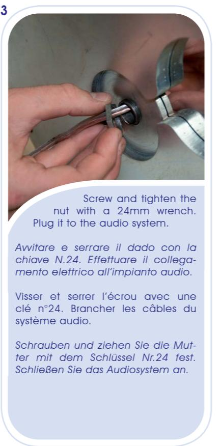
Screw and tighten the nut with a 24mm wrench. Plug it to the audio system.
